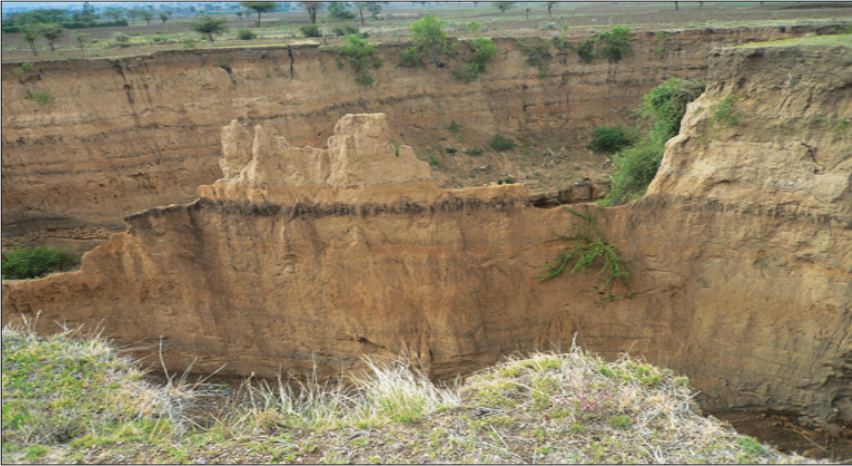
Figure 2.15: Gully erosion This very deep gully developed because of the construction of the main road at Kurfa, past Nazareth (Adama), on the way to the town of Wolenchiti, Oromia Region.
