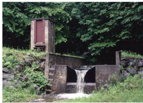
(a) Concrete dams and weirs built across streams at the bottom of watersheds enabled researchers to monitor the outflow of water and nutrients from the ecosystem.
