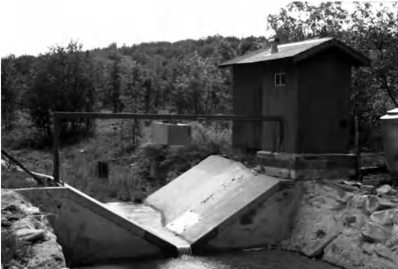
FIGURE 6.4. A broad-crested trapezoidal flume for measuring open channel streamflow
