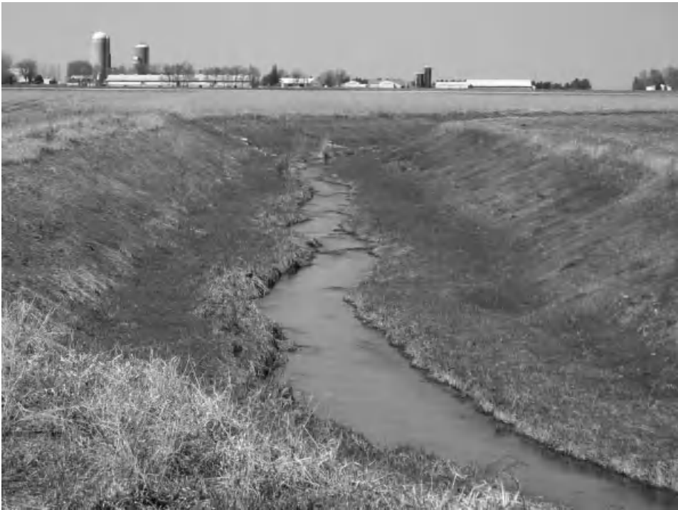
FIGURE 14.2. Two-stage ditch in southern Minnesota, USA, provides a buffer from cultivated land and roads (Photograph by Geoff Kramer)
