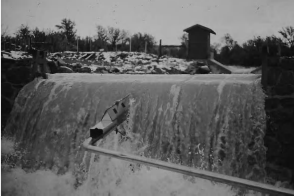
FIGURE 9.5. A sediment splitter diverts progressively smaller fractions of streamflow to a collection tank to sample suspended sediment flowing through a rectangular weir in north-central Arizona. By also collecting bedload materials that settle in the catchment basin upstream of the weir total sediment yields can be measured from a watershed (For a color version of this photo, see the color plate section)
